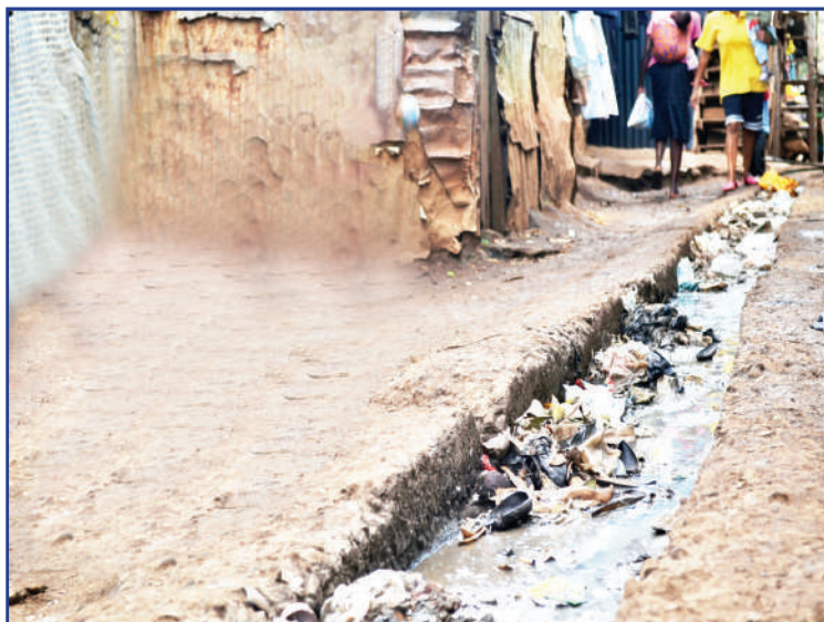
Figure 4.12: Open sewage and sanitation conditions.
